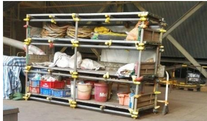
Erect Storage rack 搭建儲物架
